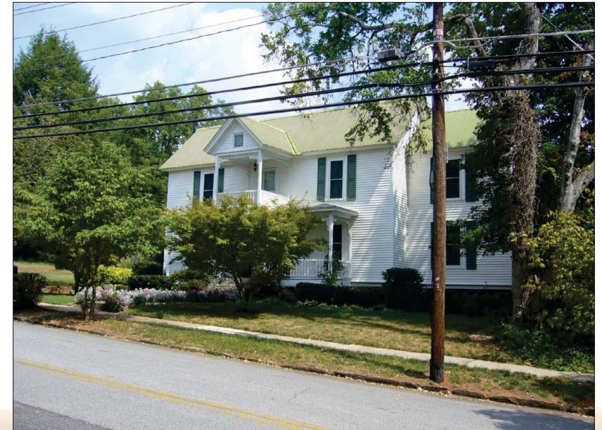
Figure 3.15: South Park Street Character
