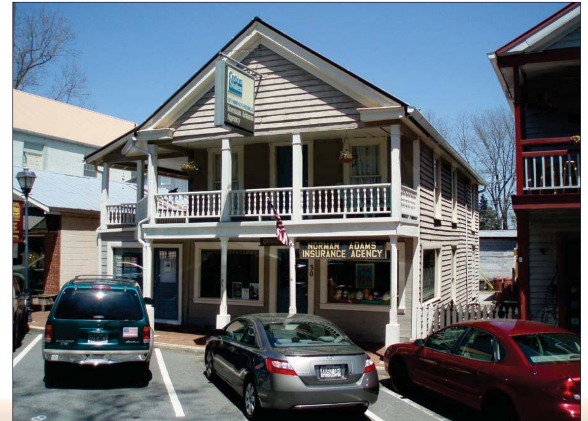
Figure 3.17: Crawford House, Public Square
