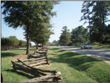
Stormwater bio-swale
