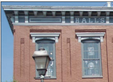
Built-up cornice on brick masonry
