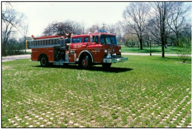
Pervious parking with "Grasscrete"
